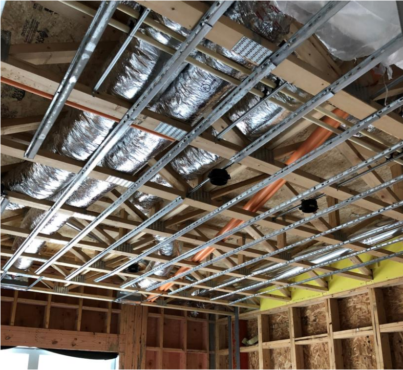
Detailing for floor/ceiling assembly
