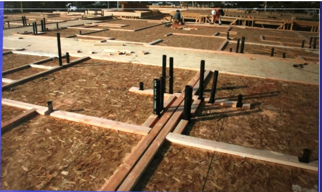
Separate Shear Walls & Plumbing Walls
