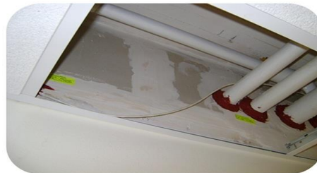
Fire-rated corridor: The way it should be
