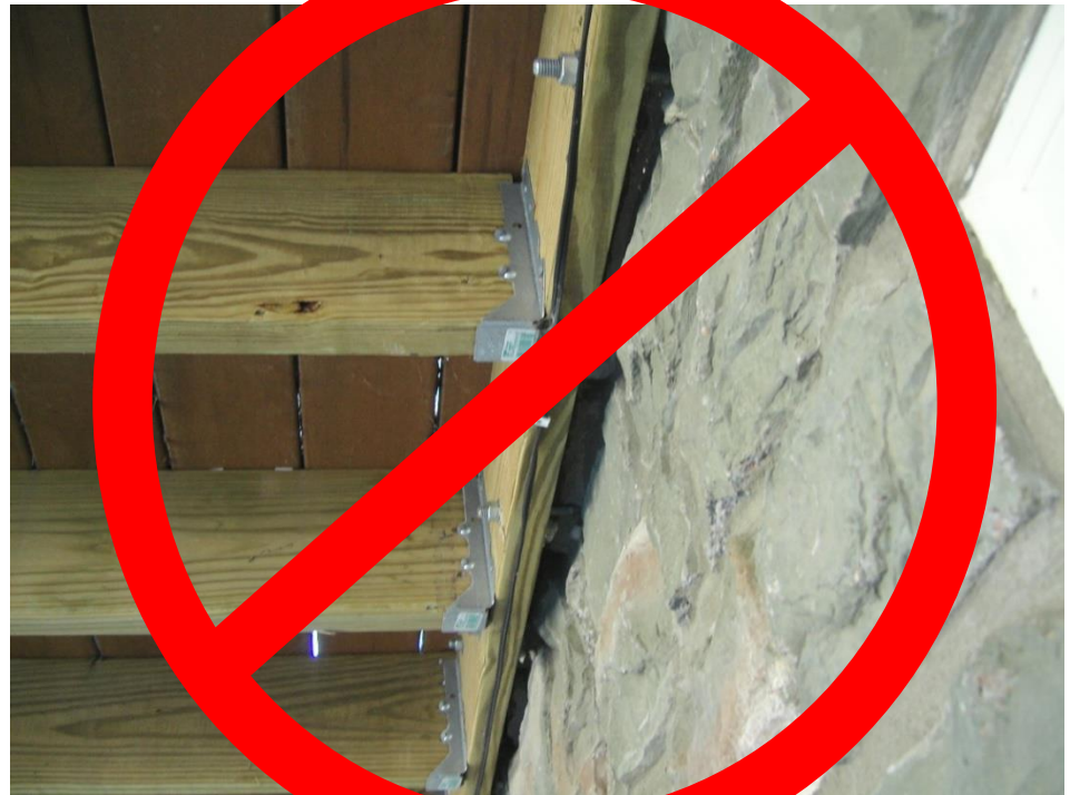
Figure 17. No Attachment to or Through Exterior Veneers (Brick, Masonry, Stone)
