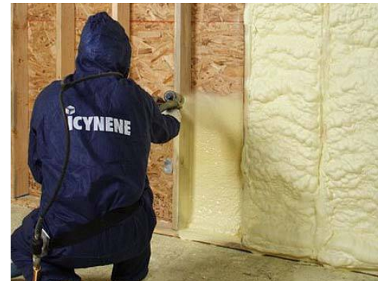
Sprayed Polyurethane Foam Open Cell/Closed Cell R = 3.5/6.0 Per inch
