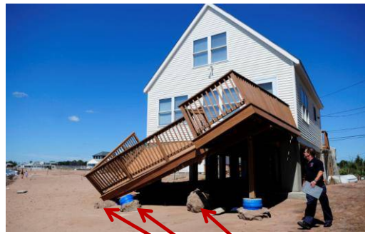
These footings appeared to have been subjected to scour or erosion from wave action
