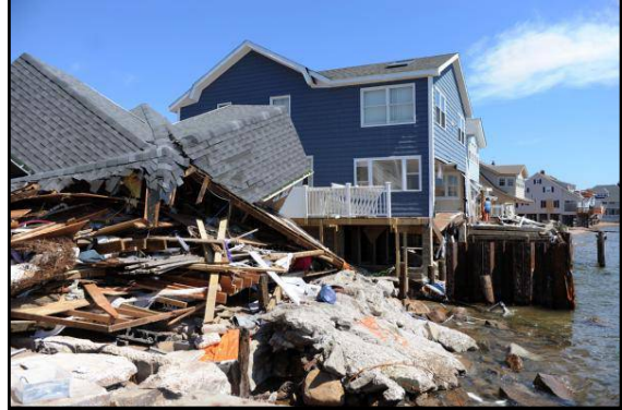
Shore Side Facing East
