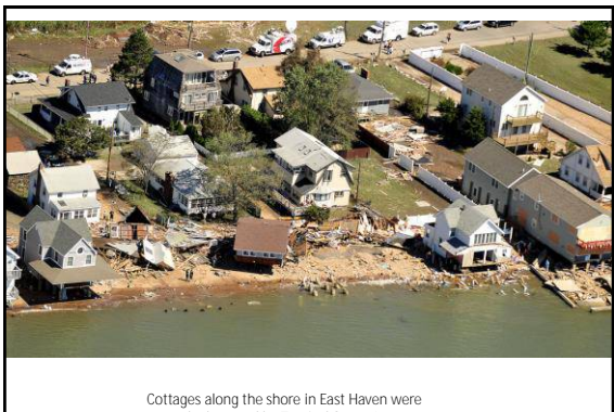
Cottages along the shore in East Haven were severely damaged by Tropical Storm Irene
