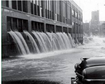
Waterbury, August 1955. Water pours from the windows of the American Brass ...
