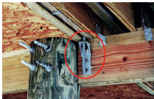
Shear wall hold down connector with bracket attached to a wood beam
