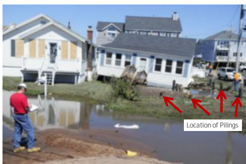
( Bettina Hansen, Hartford Courant / August 29, 2011 ) Photo taken after Hurricane Irene , Coesey Beach in East Haven. This home was swept right off its pilings.
